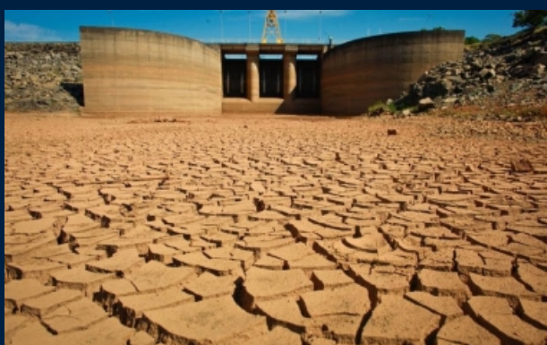
Cantareira system reservoir completely dry.
