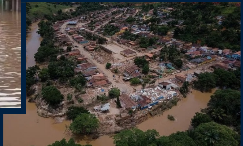
Damage caused by flooding in the Nova Alegria district after heavy rains. Photo: Eduardo Anizelli/Folhapress
